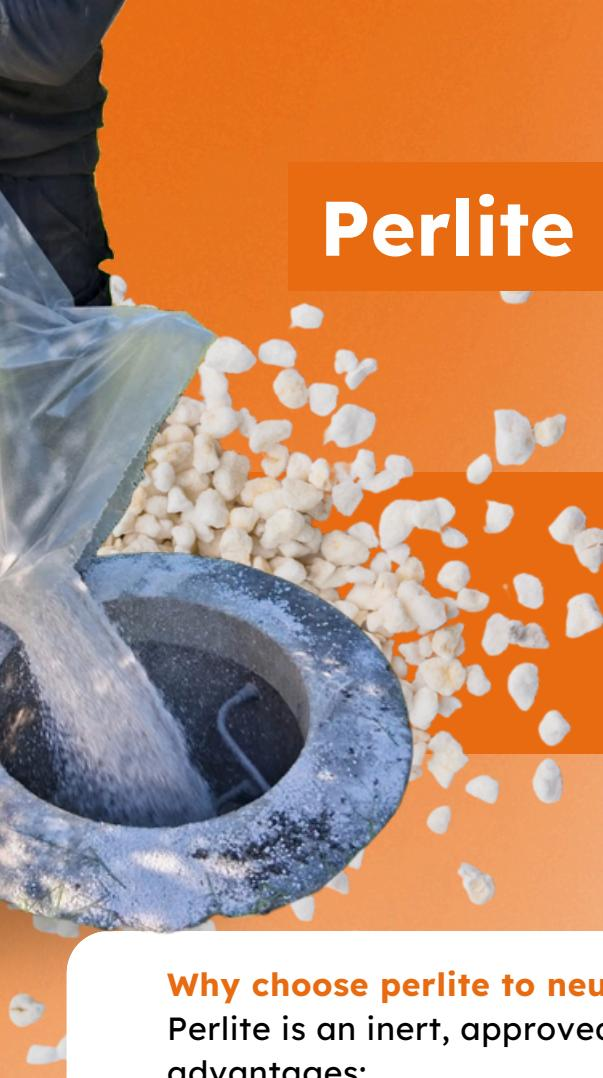
If a fuel tank cannot be removed, filling it with perlite is a simple and safe way of neutralising it.
