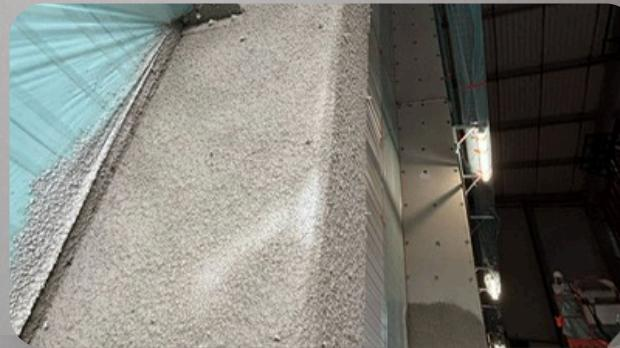
For effective fire protection inside buildings, SLV INTERNAL, a premixed sprayed mortar, is a lightweight, durable solution. Easy to apply, it combines vermiculite, cement and additives for optimum protection.
