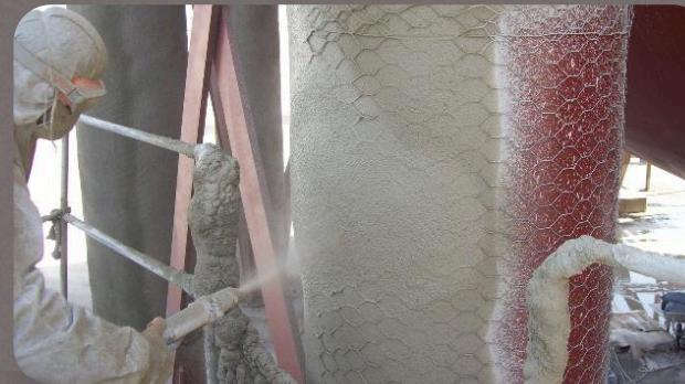
When it comes to protecting the structure of a building against the effects of a fire, SLV EXTERNAL, a premixed sprayed mortar, offers an effective solution. This lightweight mix of vermiculite, cement and additives is easy to apply and offers a durable alternative.
